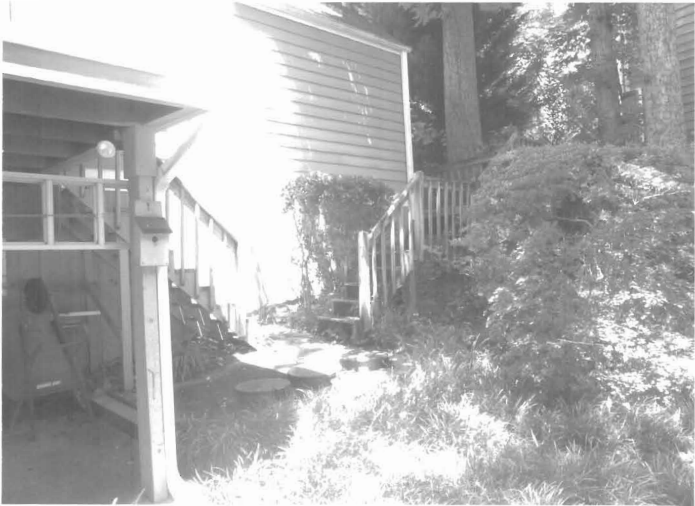
EXISTING LANDING + STAIRS
